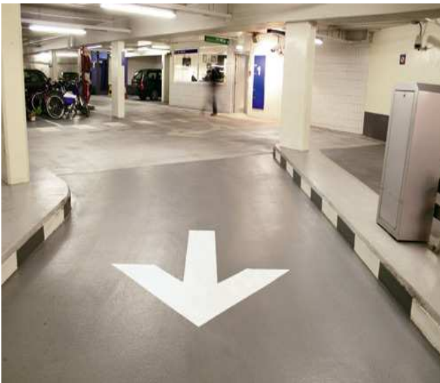
Car park flooring using Coathylene® as a structuring agent
