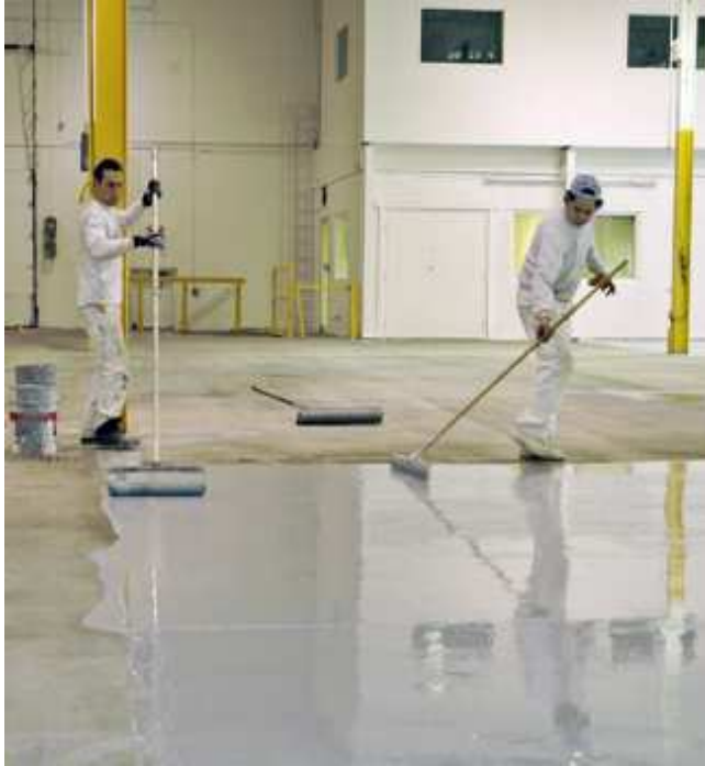
Industrial epoxy flooring using Coathylene® as a anti-slip agent
