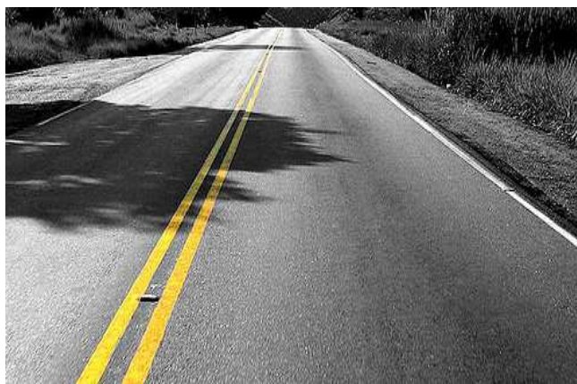
Road marking using Coathylene® as an anti-slip agent
